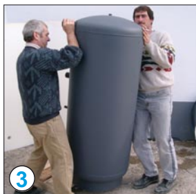
3 Lift the tank of the pallet
