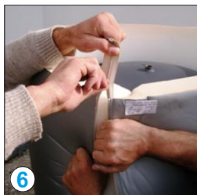
6 Watch out when closing the zipper (danger of tearing the insulation when cold) Do not use a tong or other tools.
